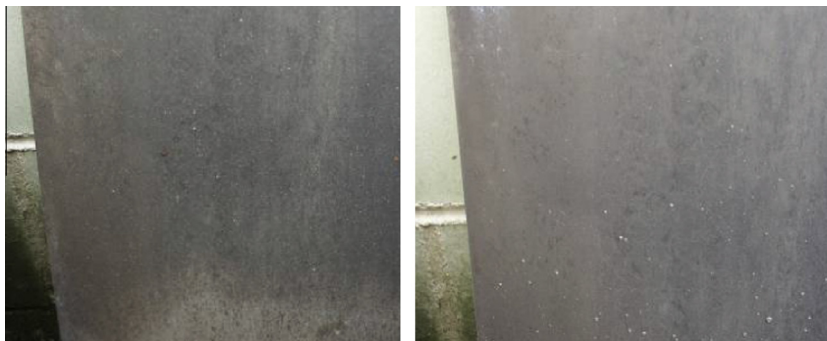
Fig. 14. Micrographs both before and after storage of sprayed oil 2.
