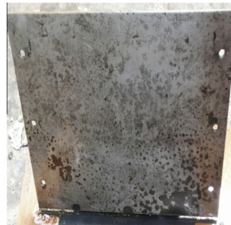
Fig. 3. Used formwork surface.
