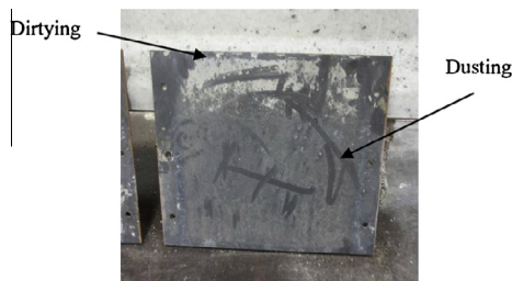
Fig. 9. Formwork obtained with vegetable oil.
