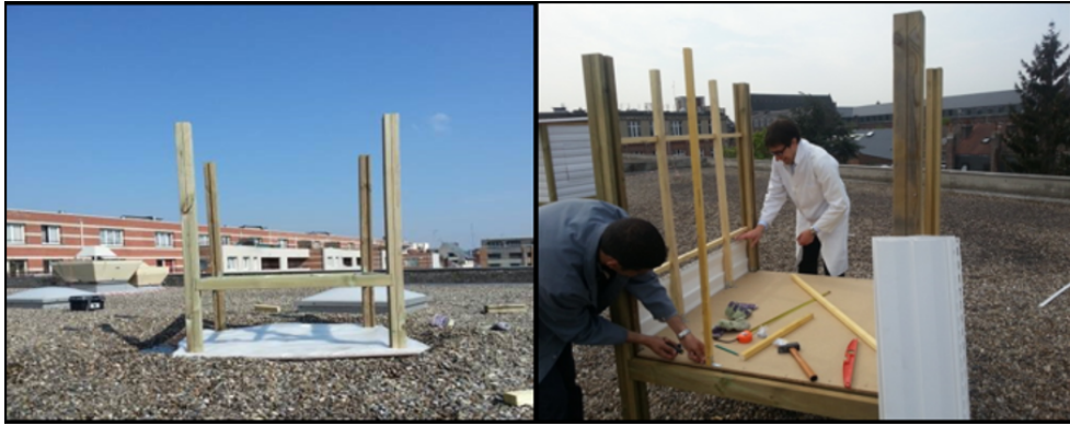
FIGURE 2.11 – Montage du box in-situ
